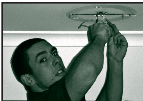
Ben repairing cables
